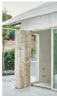
TM-01 LIGHT COLOURED TIMBER SHUTTERS
