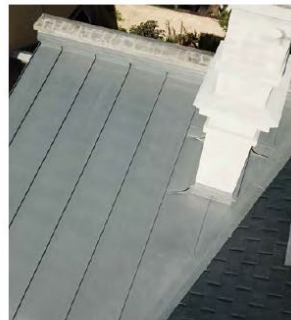
MT-01 LIGHT COLOURED STANDING SEAM ROOF
